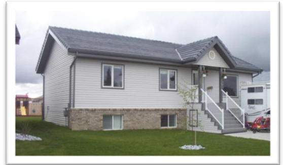
Ambrose Residence Fort St. John BC- Greensmart SIPs
