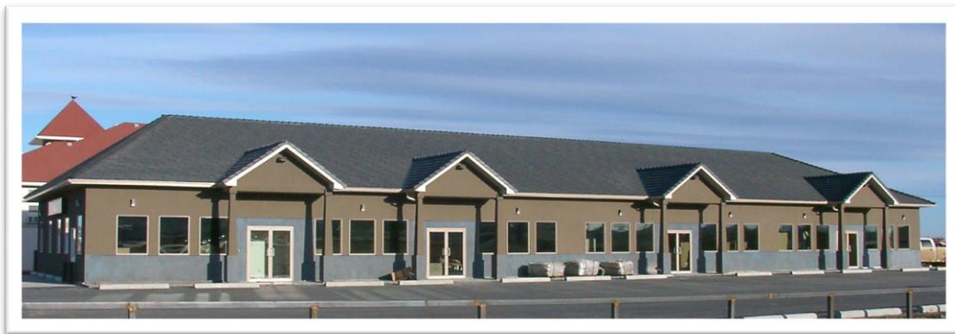
Commercial Plaza - Greensmart SIPs Dawson Creek BC
