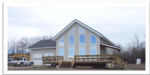
Baldonnel Home- Greensmart SIPs
