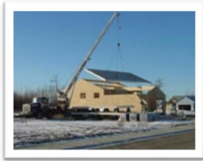
Greensmart SIP Roof Panels Fort St John BC
